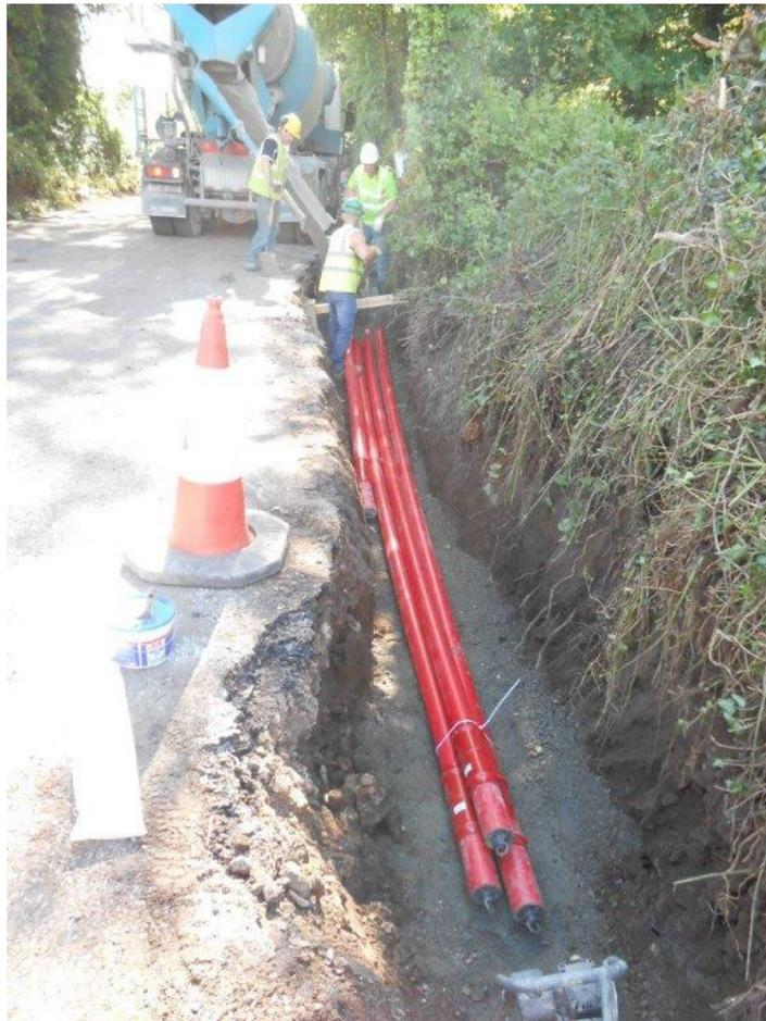
**Plate 2-1: Cable Duct Laying in Trefoil Configuration**
